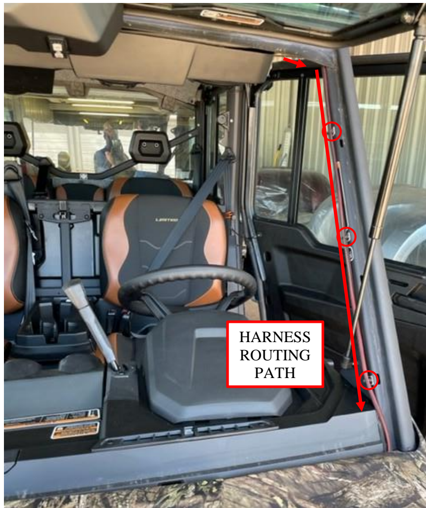
Figure 24: Route the chassis harness down the driver's front pillar.
